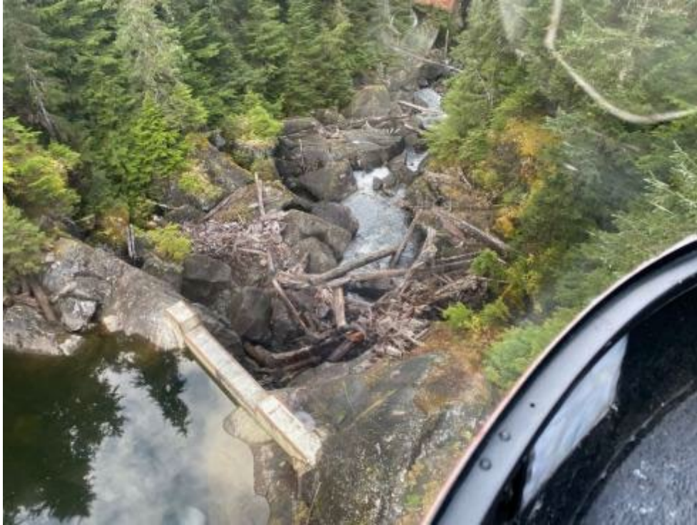
Photo 5-1 Tyee Creek at the Tyee Lake outlet weir looking downstream when no water is flowing from Tyee Lake over the weir.
