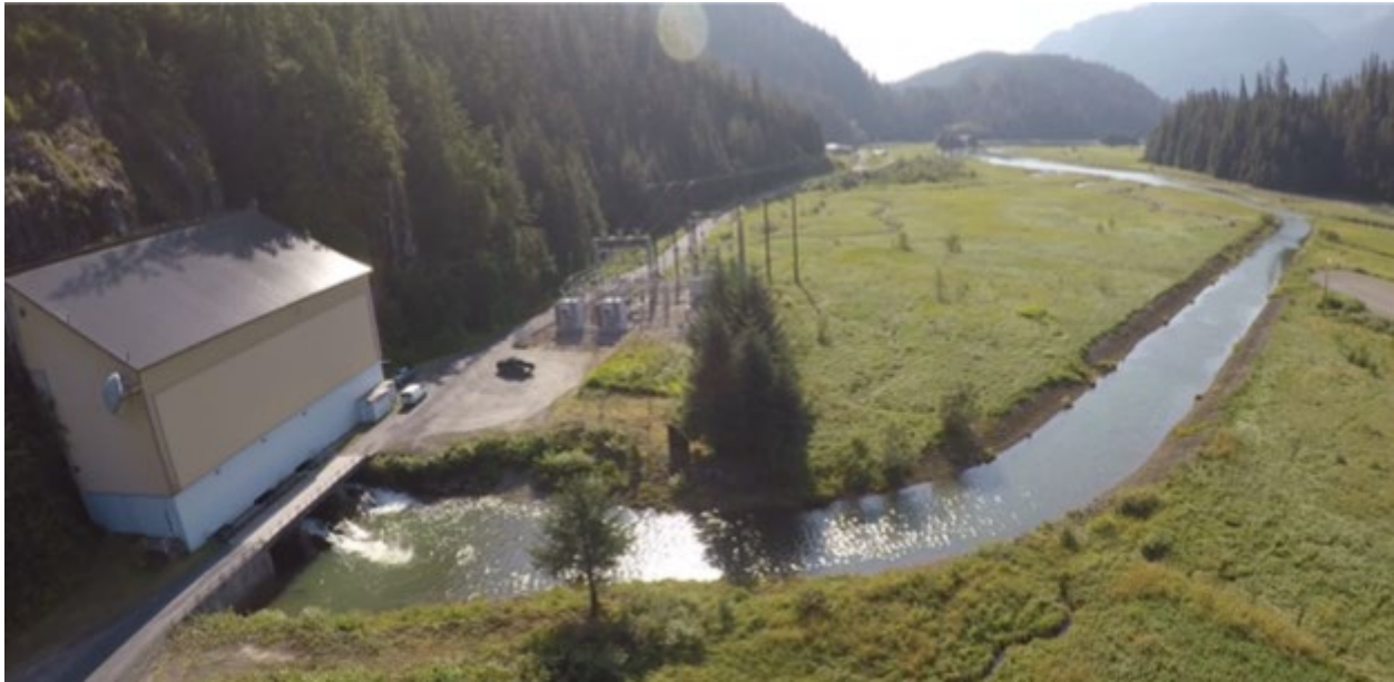
Photo 3-4 Tyee Lake powerhouse, switchyard, and tailrace.
