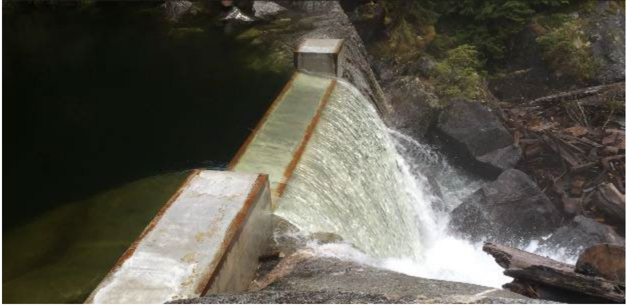
Photo 3-2 Tyee Lake spillway weir.
