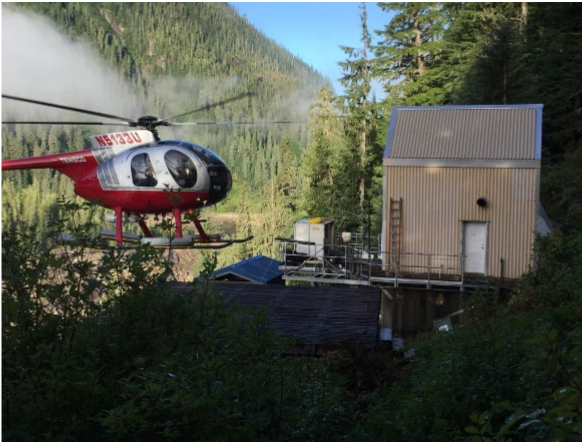
Photo 3-8 Gatehouse at Tyee Lake.
