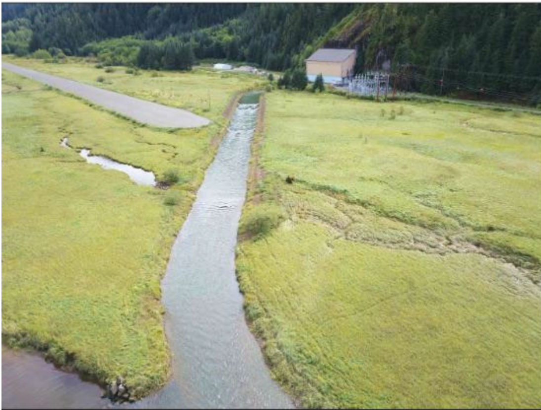
Photo 3-6 Tailrace looking upstream from Airstrip Slough to the Tyee Lake powerhouse.
