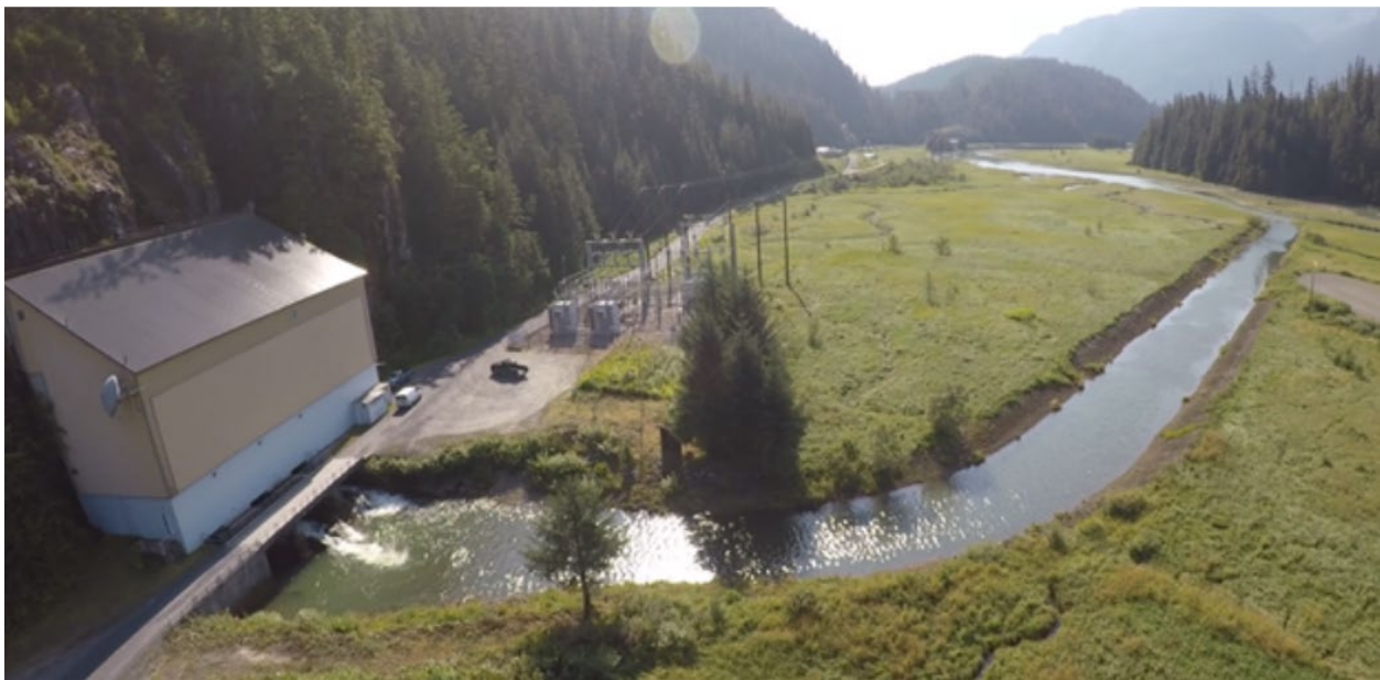
Photo 2-2 Tyee Lake Powerhouse, Switchyard, and Tailrace.
