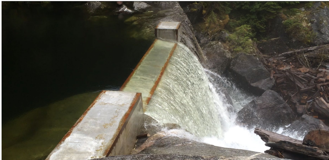
Photo 2-1 Tyee Lake Spillway Weir.
