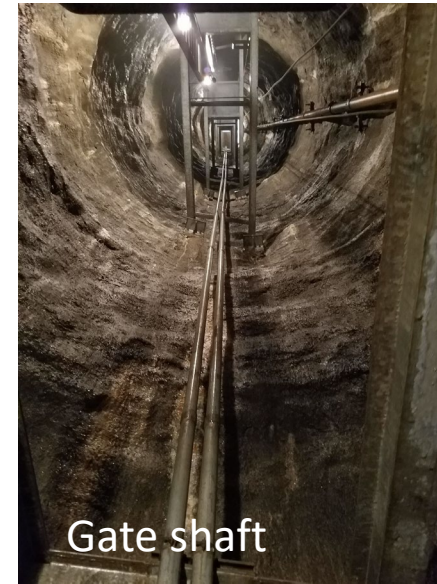
Gate shaft intake gate
